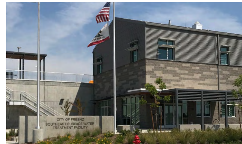
The recently completed City of Fresno Southeast Surface Water Treatment Facility is actively contributing to meeting the water usage consideration goals of the Blueprint.
